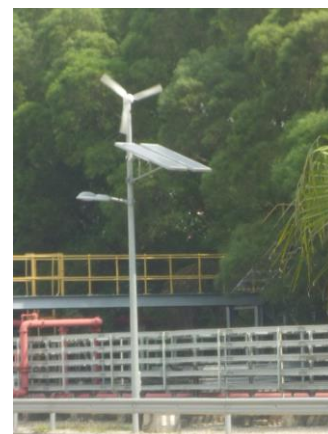
Lamp Driven by Wind Turbine and Solar Panels at Black Point Power Station
